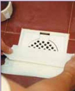
Seal off all gully and floor traps.
